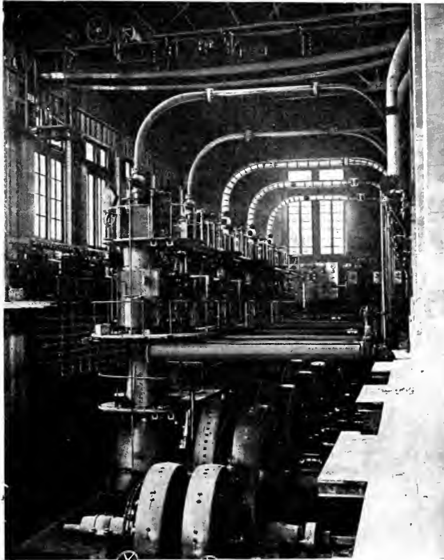
FIG. 1.—VIEW OF ENGINE ROOM.
